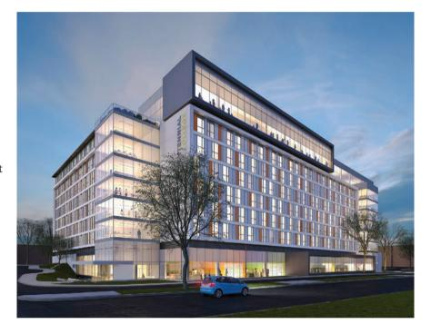
structural steel for the larger columnfree spaces, and flat plate concrete construction on the residential floors.
